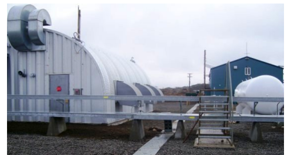
Building which houses the hydrogen genset
