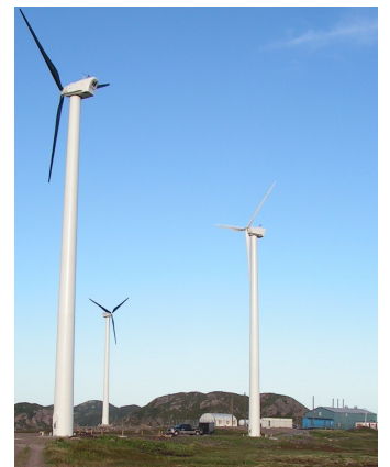
Northwind 100B 100 kW turbines
